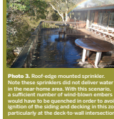
Photo 3. Roof-edge mounted sprinkler. Note that the sprinklers did not deliver water to the near-home area. With this scenario, a sufficient number of wind-blown embers would have to be in this zone, particularly at the deck-to-wall intersection.
