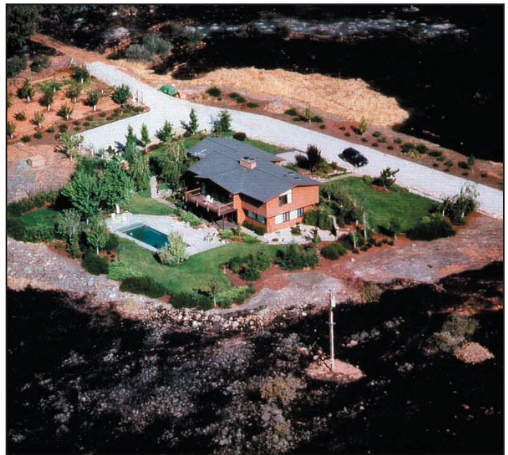
The pre-fire activities implemented by this homeowner included a green and well maintained landscape, reduction of wildland vegetation around the perimeter of the property, a fire resistant roof and a good access road with a turnaround area. As seen in this photo, these pre-fire activities were effective.
